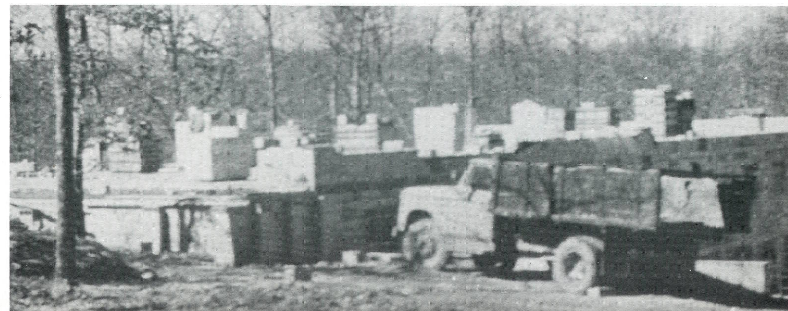
The Vocational Arts Building (under construction)
