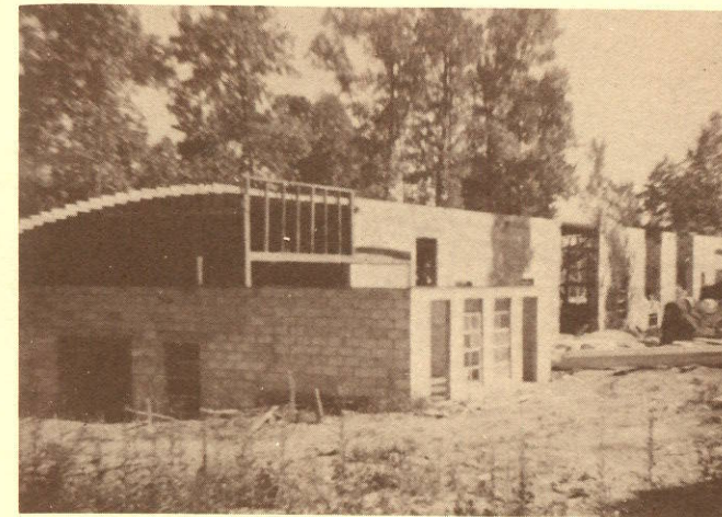
Building the Shop
