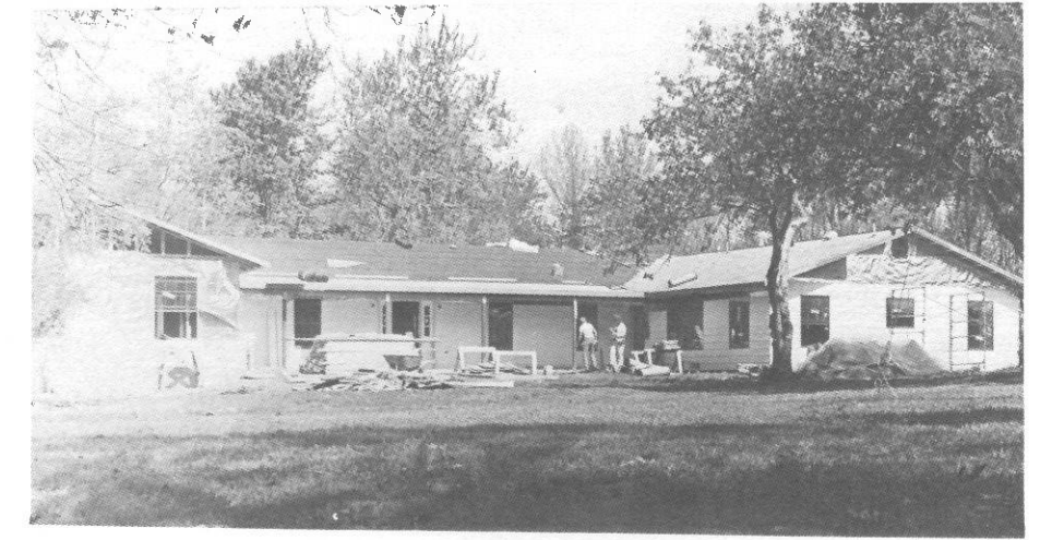
The building on April 25
