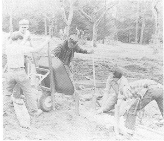
Pouring the footing
