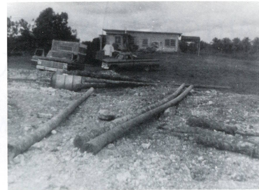
Poles for the Shop
