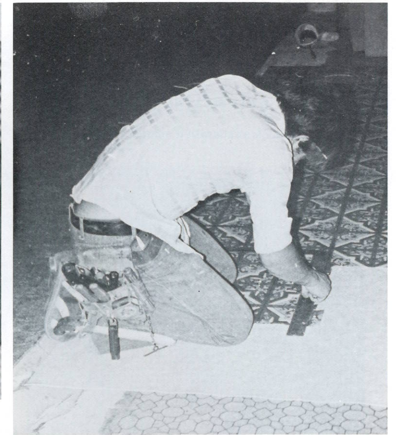
John putting down new flooring for the lounge room
