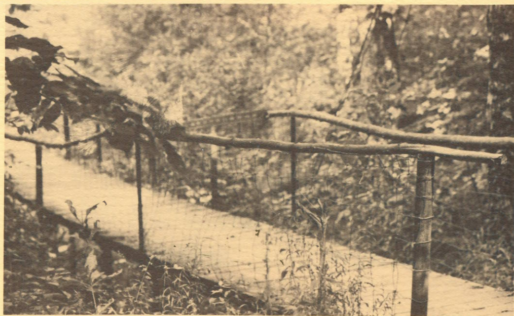
The Bridge Each day we pass here to and fro. . . to cross the creek that's down below.
