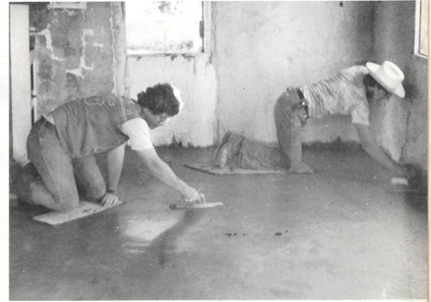
Mark and Duane troweling.
