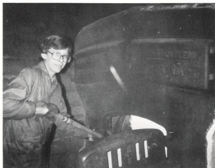
Steve Fires the San Boiler
