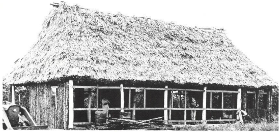
Building a new clinic
