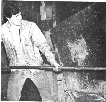
Dan will show you how to fire boiler
