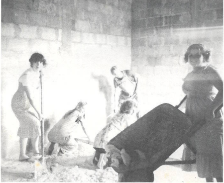
Floor laying crew.
