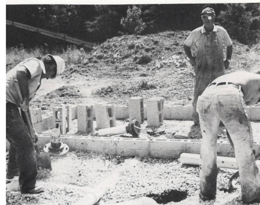
Mr. Schoonard lays out the barn.
