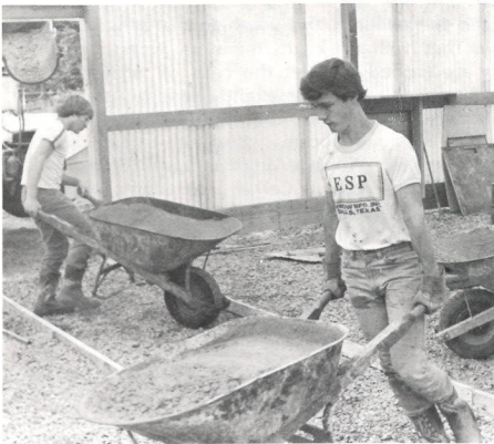
Building the Greenhouse
