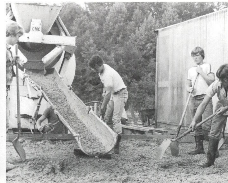
Learning Cement Work
