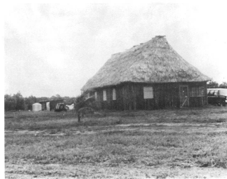
The Medical Clinic Which Is Typical of the Buildings There
