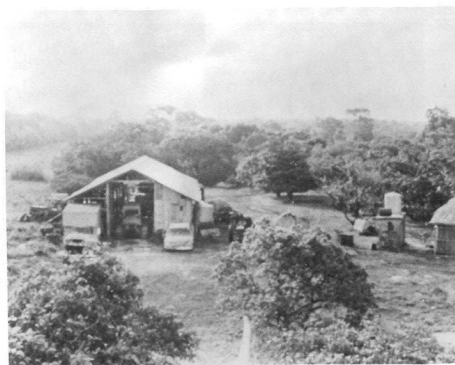
Their Shop Building Which Laurelbrook Helped Construct Several Years Ago
