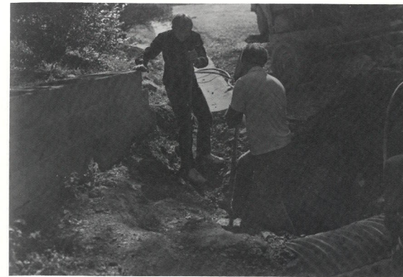
Just one more shovel of dirt!
