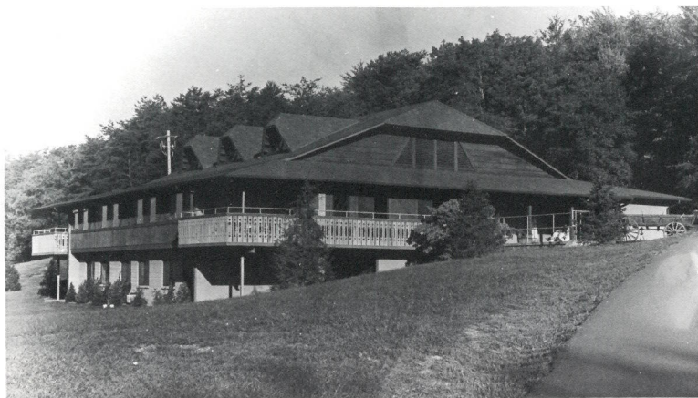
This is the main building at the Cohutta Springs Camp.
