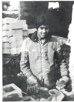
Priyason works on coal bin.
