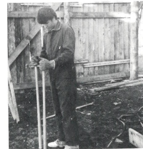
Jeff digs postholes for the new barn.
