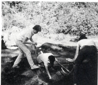
Sophomores dig a water line ditch.
