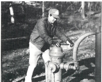
Arturo cleans out fire hydrant.
