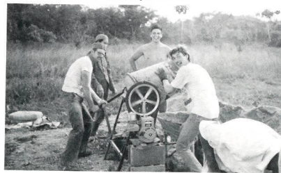
Mr. Ellis, Dan, and Tom mix cement.
