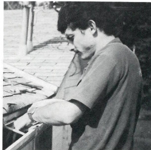
Alfredo works on the Center Building roof.
