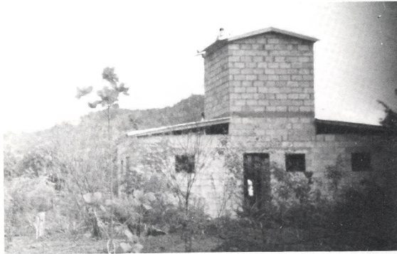
Now the bathhouse and water tower are almost completed.
