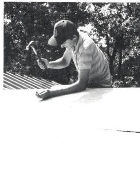
Seth works on the dorm addition.
