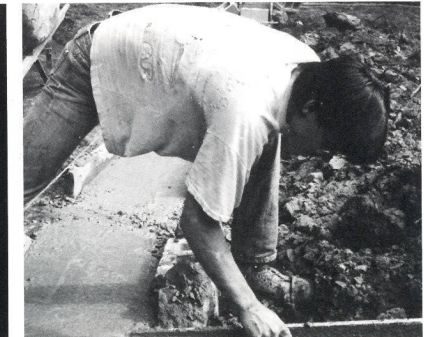
Tom carefully smooths the cement.
