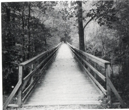
This bridge crosses the creek to our chapel.
