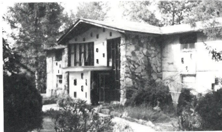
This is the ad building and cafeteria.
