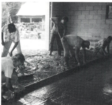
Construction lays the fire house floor.
