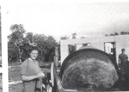
Sonya operates the cement mixer.
