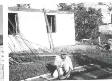
Jamie cleans cement off the wall forms.
