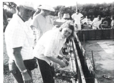
C.D. Carter and Sonya set up the cement wall forms.
