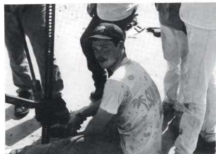
Todd digs out a stump in the foundation.
