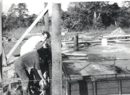
Cheri and Jennifer set up the first level of the wall.
