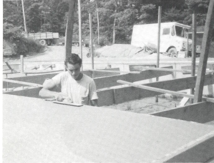
Richard skillfully smooths out the cement.
