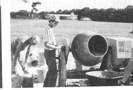
Seth operates the cement mixer.
