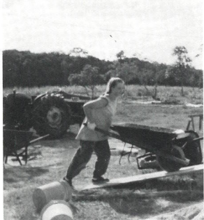
Sylvia pushes a wheelbarrow up the ramp.
