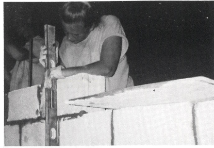
Sylvia Huckabee makes sure the wall is straight.
