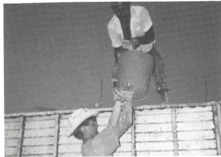
David Norman hands up a bucket of cement to be poured.
