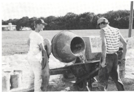
David Norman operates the cement mixer.
