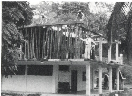
Our project was to build a second story above the cafeteria.
