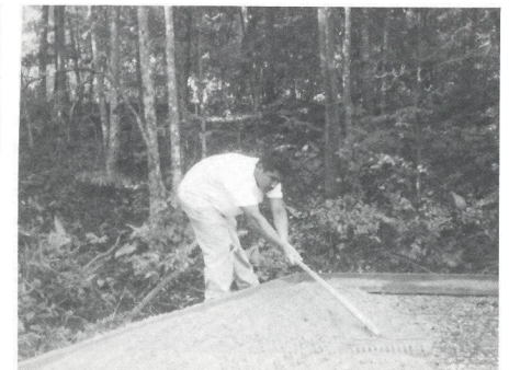
Ron spreads out the concrete for the gas pump pad.
