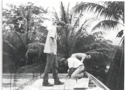
Matt, Hector, and C.D. work on the roof.
