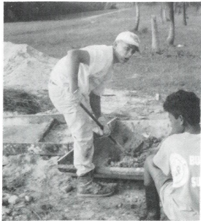
Teddy supplies the workers with cement mix.
