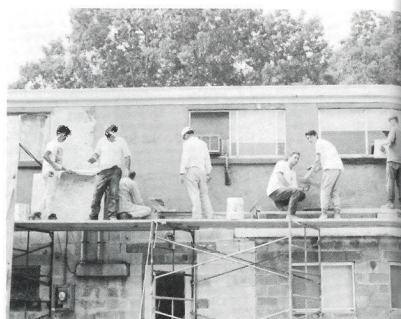
The boys work hard trying to cement the wall.
