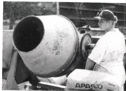
Kelley energetically runs the cement mixer.
