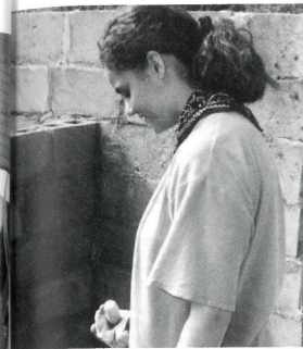
Sarah tries to hide while laying a block wall.
