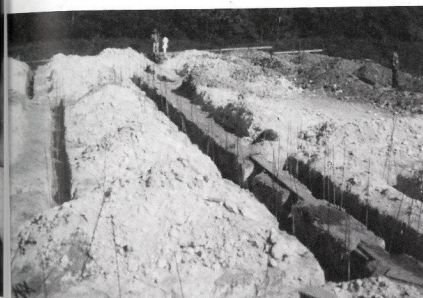
The work site.
