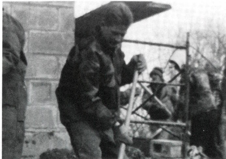
Jeremy digs ground for Mrs. Wellman's house.
