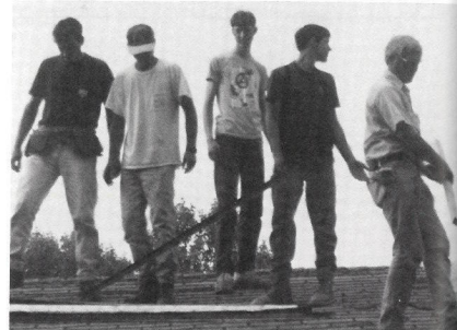
Mr. Schoonard instructs the boys about roofing.
