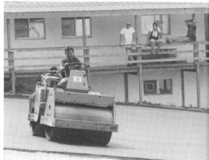
The paving begins.
