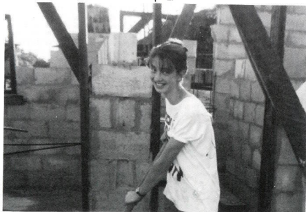
Rachel mixes up cement for the PVHI shop building.
