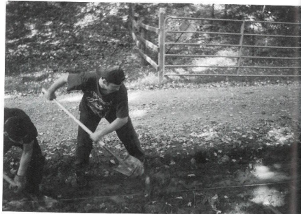
Gary digs a ditch.
