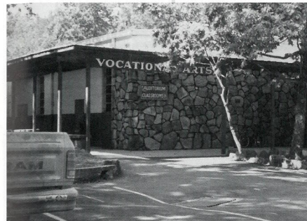
This is our VA Building (classrooms) and auditorium.
