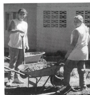
Janelle and Michelle J. get introduced to mixing concrete.
