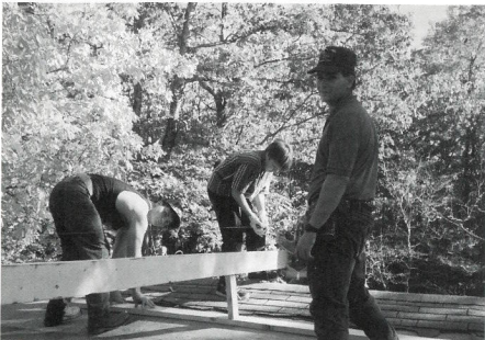
J.R. helps with building the addition on Mr. Eric's house.
