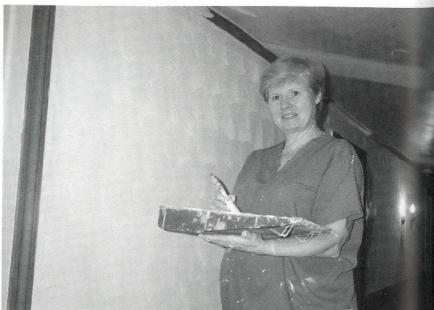
Mrs. McDonald stuccos the walls in the girls' dorm upper hall.
