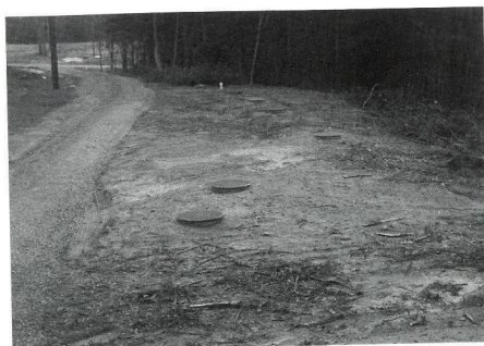
New pipes and holding tanks for the waste water system behind the nursing home.
