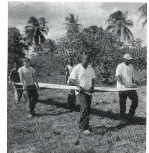
Kendrick, Steve, and Warren carry some metal roofing.
