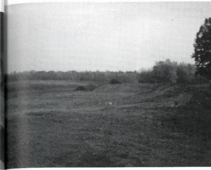
This is a view of the new irrigation pond.
