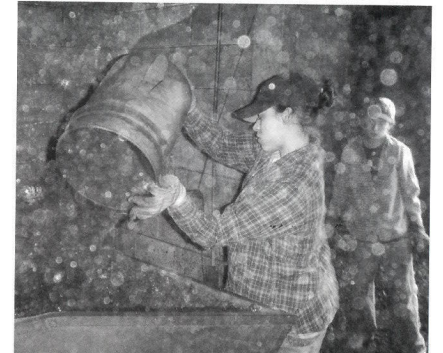
Patricia loads the coal hopper for the grade school boiler.
