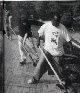
Tim and David Parnell scrape off the old shingles on Mr. Joel's roof.
