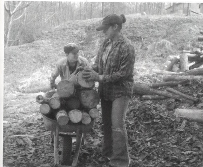
The girls haul in the wood for the main school boiler. At this time, the coal mechanism had broken down, and the boiler was being heated with wood.
