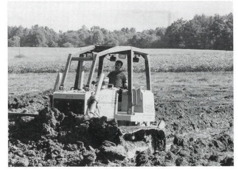
Mr. Rodney works on excavating the new pond.
