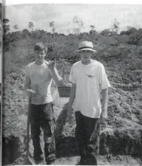
Kendrick and Tim take a breather from digging the footing.
