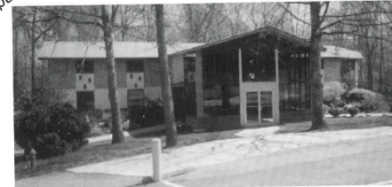
We've made progress on the addition to the administration building - a new lobby.
