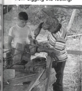
Kendrick and Mr. Bob prepare reinforcing steel.
