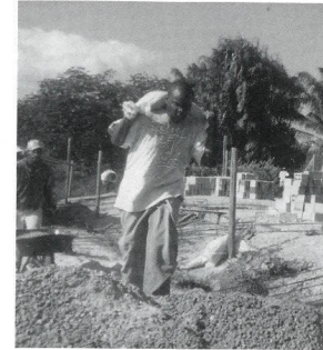
Dump truck David is about to unload some gravel.
