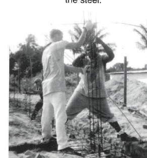
Andy and David make sure the building stays put.
