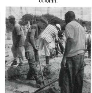
Kendrick shows Steve how to mix cement on the ground.
