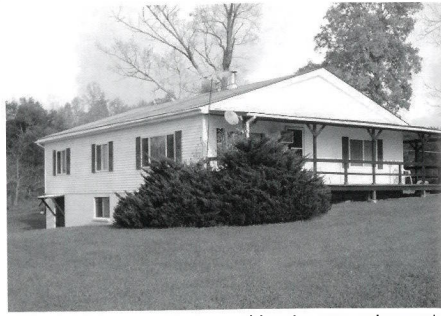
Wendel Adams and helpers did major renovation work on this house near the cemetery.
