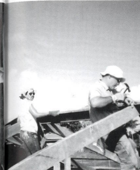
Mr. Chuck and Raquel nail on the roof beams.
