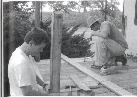
Mr. Mario and Jonathan work on the Baileys' house.
