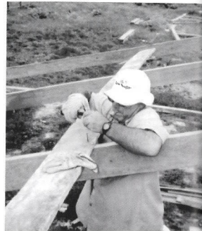
Mr. Chuck skillfully builds the roof.
