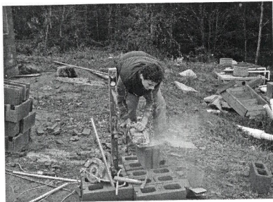
Matthew cuts block for the walls of the new waste water plant.
