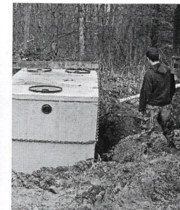
Ben watches the septic tank ease into the hole he helped dig.
