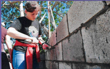
Leilani scrapes off excess mortar from the wall.
